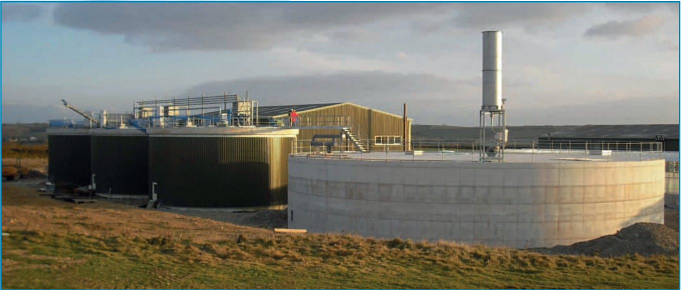
Biogasanlage Langage Farm, UK – Plymouth: 12.000 t/a Speisereste, 3.000 t/a Gülle
