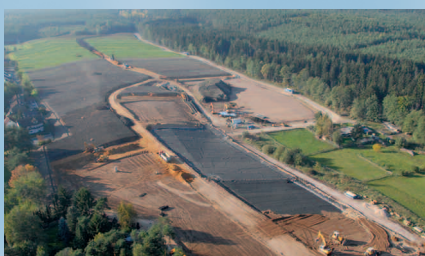
Landfill under construction
